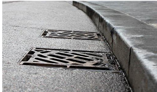
Fig. 7.7 Trapped road gully
