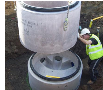
Fig. 7.5 Precast concrete ring manhole (reproduced from Woolley 1988 with permission of E & FN Spon)
